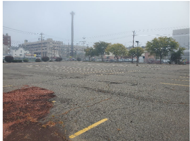
Looking northeast across site. Note existing parking structure in background.
