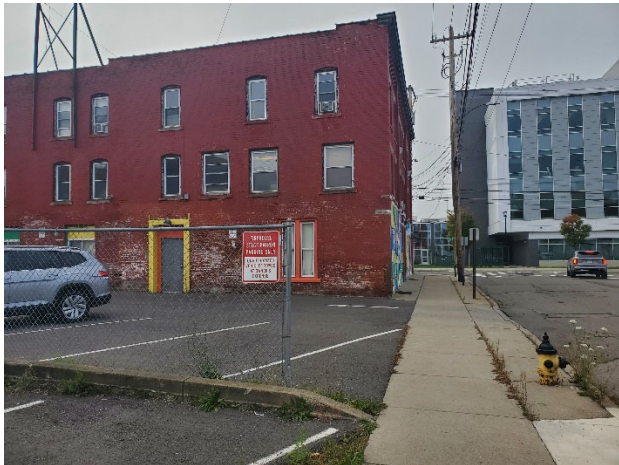
Looking south at theater building. Note side yard distance along Broad Street. Binghamton University building in background.
