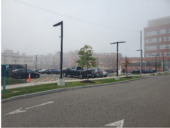
Looking southwest across site.
