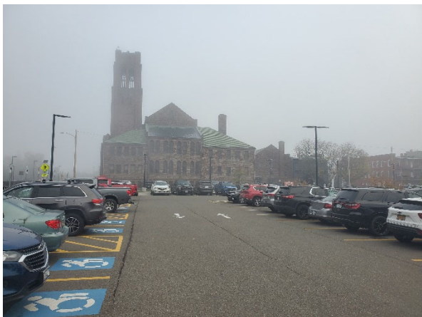
Looking north from southern parcel line.
